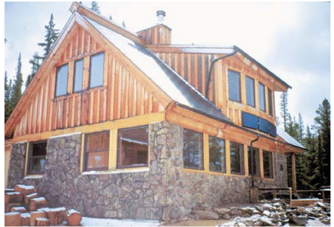
Above: The Traditional style of Uncle Bud's Hut integrates perfectly with the natural beauty of the Rocky Mountains. Notice the winter oriented (vertical) array before its replacement with an all-season pole mount system.
