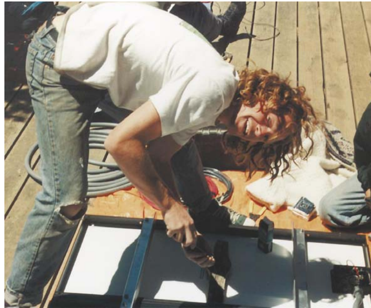
Joe Schwartz, an SEI student, wires the replacement panels for pole mounting at Uncle Bud's Hut.
