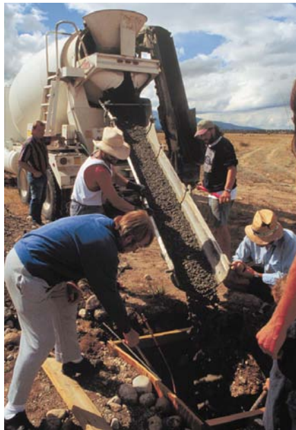
Above: Pouring concrete for the footings.
