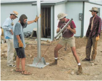
Leftt: Installing ground rods. Author Logan Brown stands at far right.
