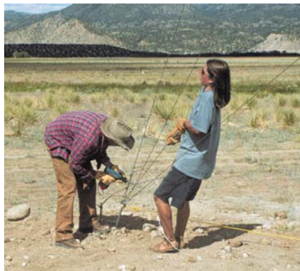
Below: Tensioning the guy cables.
