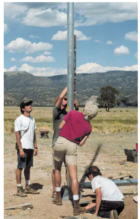
Right: Making sure the tower is plumb.
