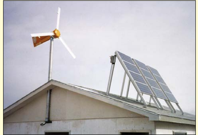
The original Bergey "tower"
