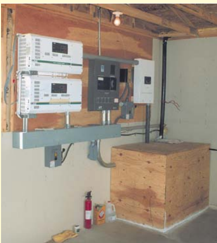
Left: The control room in the garage. Note the "safety equipment" on the floor.
