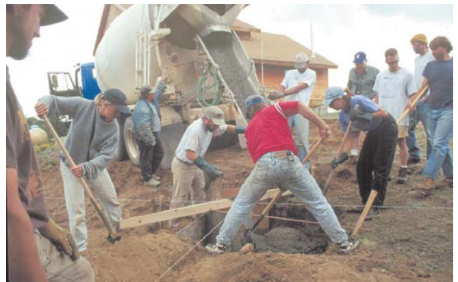
Pouring concrete for the tower anchors.
