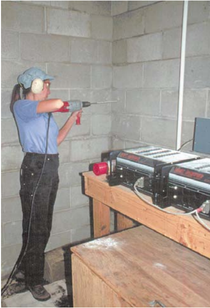
Drilling the battery room walls for tower wiring access. Note the original location of the inverters over the battery box.
