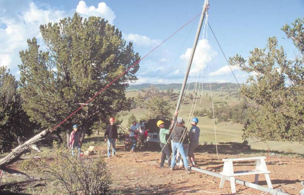
“Heave-ho”ing the tower gin pole into place.
