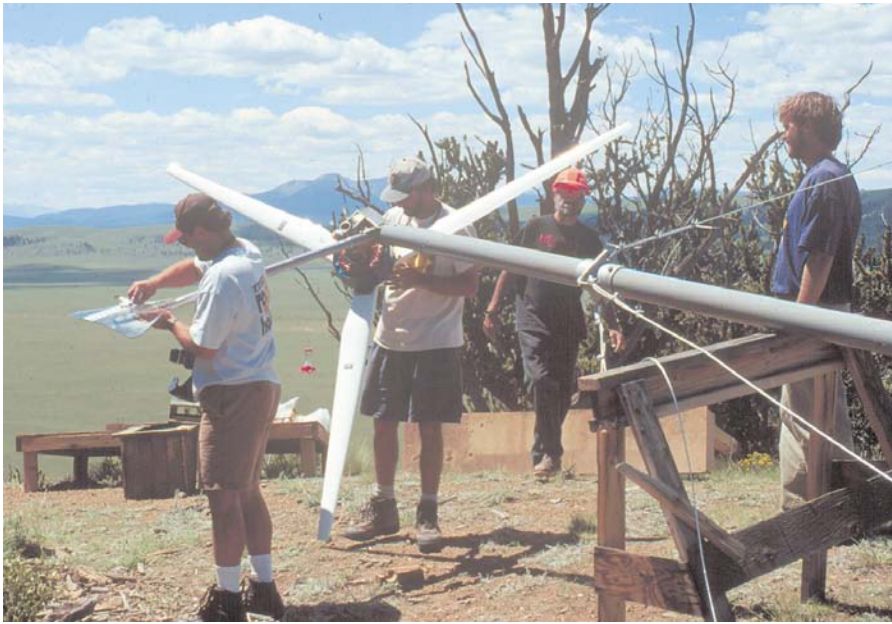
Final nuts and bolts check on the Whisper H1500 before we raise the tower.
