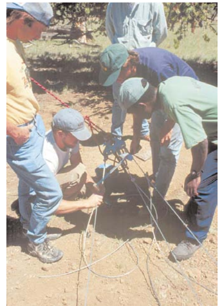
Untangling the maze of tower guy cables.
