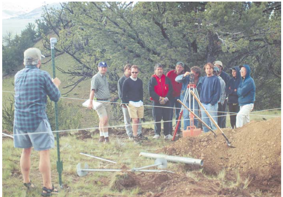
Johnny Weiss holds a makeshift surveyor’s staff while the crew checks anchor heights with a transit.
