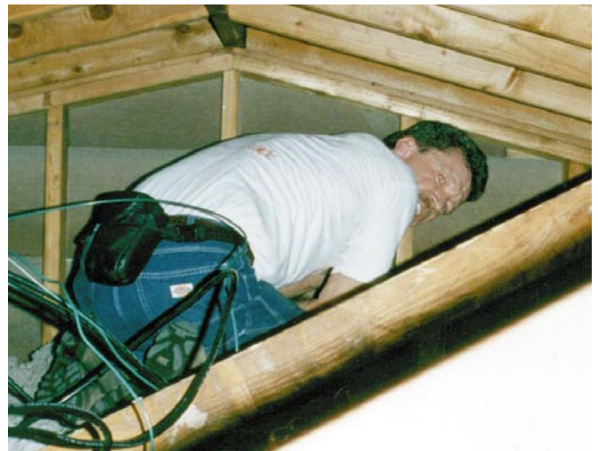
Above: Joe Flake of Go Solar Enterprises runs PV cables through Jane's attic. It is often small matters such as wiring that are critical and difficult. The hands-on training offered by SEI in their on-the-job courses gives their students experience in details such as safe and standard wiring practices. Classroom training is fine and necessary, but it must be backed-up with actual installation experience.
