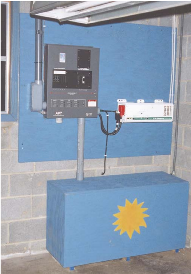
Above: The Ananda Power Center, the Trace inverter, and the vented battery box (with the yellow sun). All these components are safely and neatly installed in Jane's basement
