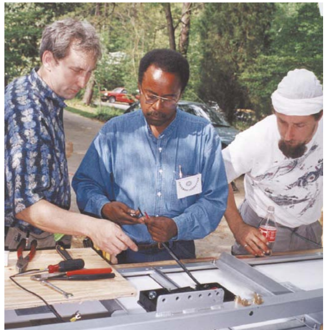
Above: Chris Carter of Solar Village Institute teaches the class how to properly mount and wire the photovoltaic array. Since PVs will easily produce power for over ten years, details such as module wiring are critical if the array is operate for ten years without problems.
