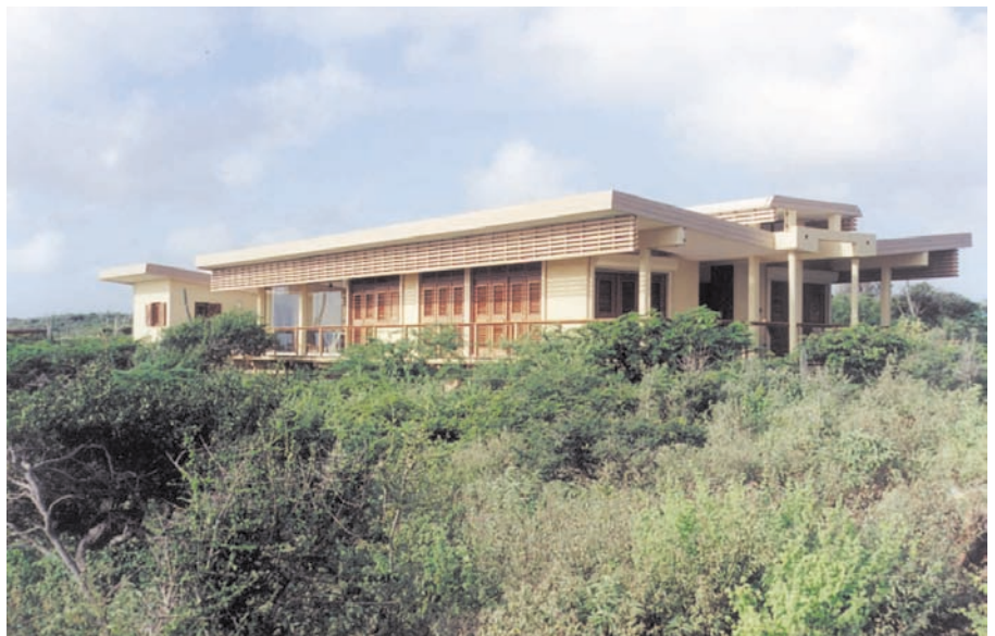
Shade/rain drop-down louvers, decks, and fascia are recycled plastic lumber chosen for resistance to climate and insects.
