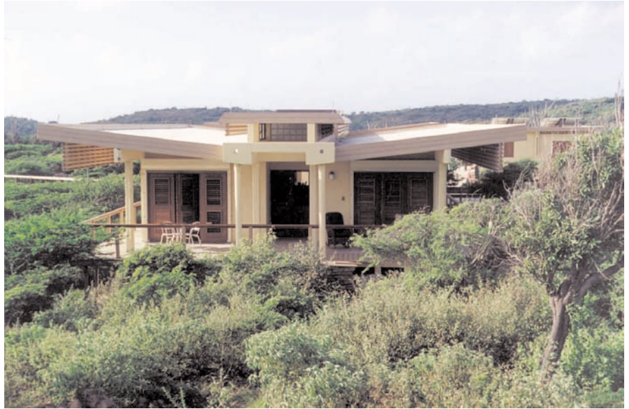
The “butterfly” roof collects water in the center, and drains it down the end columns for storage until needed.
