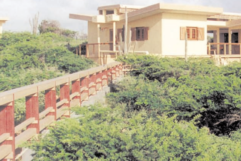
Covered water pipes (left) lead to the island house from the Southeast.
