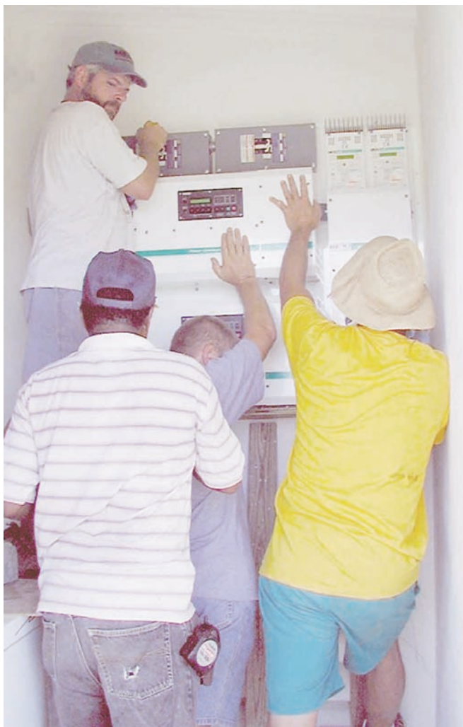
Dual Trace SW5548 inverters make mounting the power panel a group effort.
