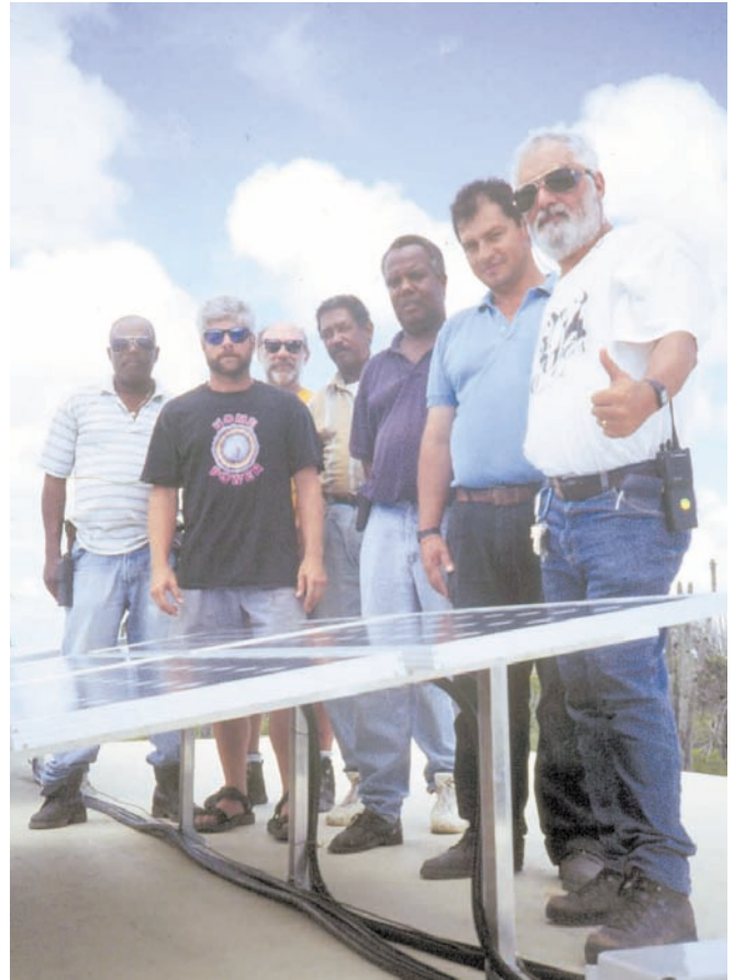
The muscle (and brains) behind the completed photovoltaic installation.
