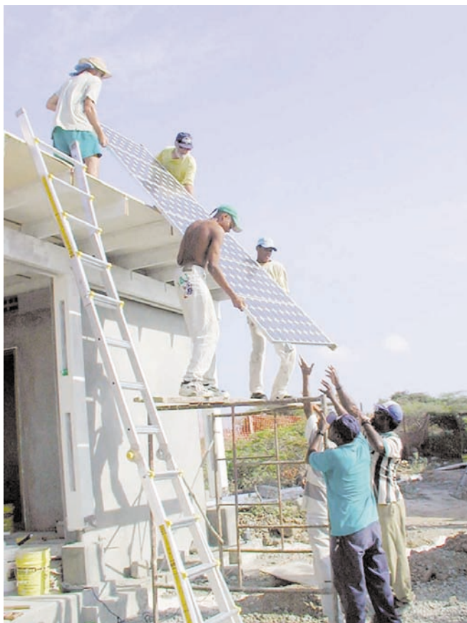
Sub-arrays were assembled in the shade, then hoisted to the roof.
