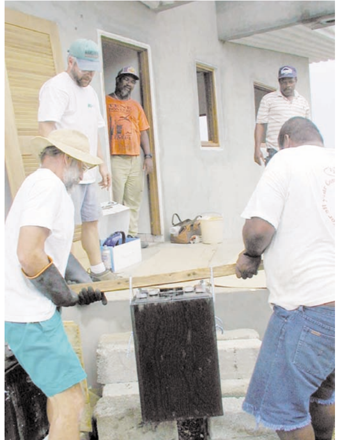
Two huge Yuasa HUP 2 volt lead-acid cells are lifted to the power room. Total battery capacity is 1,275 AH at 48 VDC.
