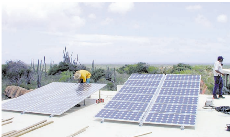
Twenty-four Siemens SP-75 PVs provide 1,800 watts.
