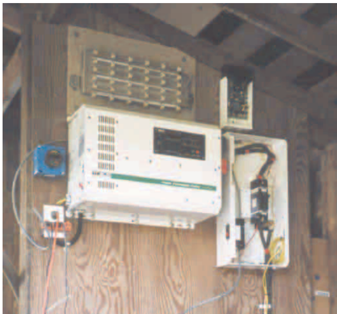
The inside of the power shed, showing inverter, DC disconnect box, charge controller, and dump load.
