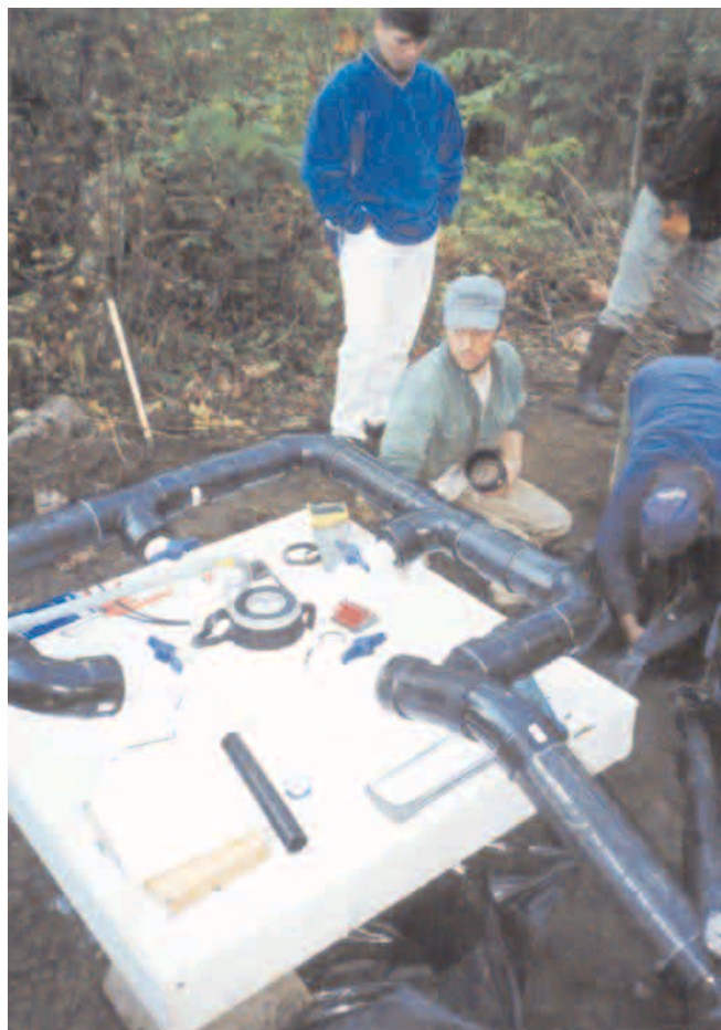
The completed manifold with the ES&D turbine.
