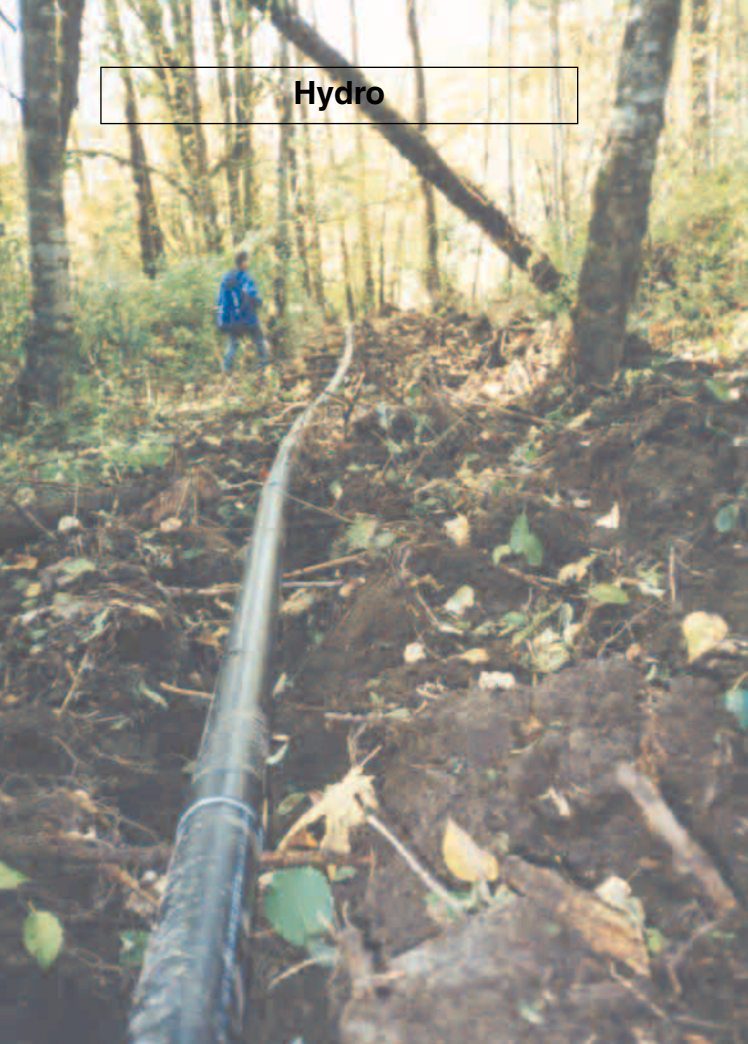
The penstock, still propped over the ditch for ease of gluing, snakes its way down to the turbine.
