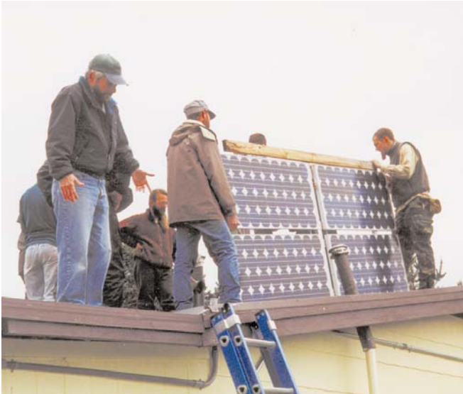
The fun part—puttin' panels on the roof.
