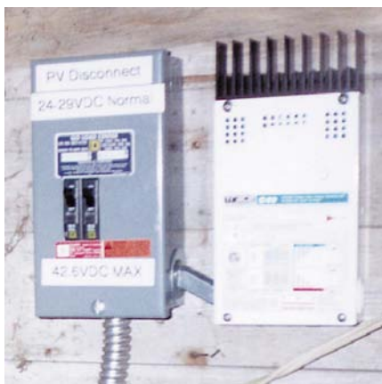
Left: Trace C-40 charge controller and bracketing 15 Amp breakers.
