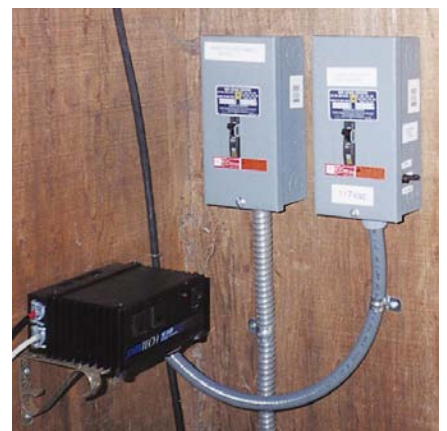
Right: Exeltech 500 watt inverter, breakers, and utility/battery switch.
