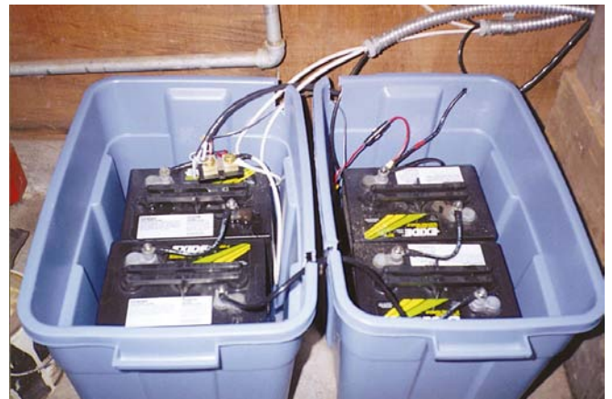
Below: Exide T-105s in spill-proof tubs.
